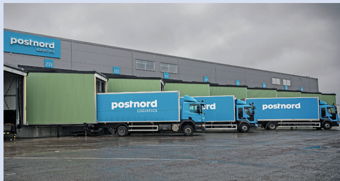
Postnord has developed a security strategy with advanced surveillance solutions to protect its assets.
