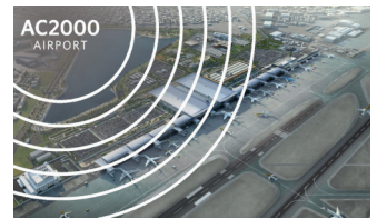
The aviation specific CEM Systems AC2000 Airport access control solution has been selected to secure the new Bahrain International Airport.
