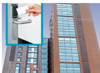
The Chamberlain student accommodation at Edgbaston, Birmingham University, secures access with Aperio.
