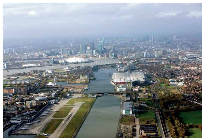
At London's Excel from 21–23 June, Ifsec International 2016 will be a strategically significant platform to present current technologies and research to the market as security systems and services play an increasingly vital role in building automation.
