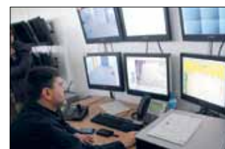
Each of the four operators works with six screens and uses the Bosch Video Management System.
